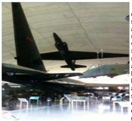
craft at Duxford. It was designed by Sir Norman Foster and had to be big enough to swallow the B52 with its 185 ft wingspan and a tail that is over 50 ft high. The roof was designed to support suspended aircraft of up to 10 tonnes so had to be substantial, yet still look good. Apparently there are 6000 tons of concrete in it. so I think you can get the general idea. As if that wasn't enough the building has a glass front facing diagonally
